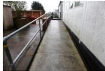
Surfaces such as hardwood or nylon coated steel are recommended in preference to surface materials that are cold to the touch. The handrails are easily distinguishable from their background, without being highly reflective.
