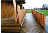
5.2 Ramps should have the following dimensions: 1.5m wide with a minimum unobstructed width of 1.5m.
