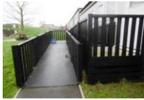
Not all of the ramps have handrails on both sides. Normally people who have difficulty negotiating changes of level need the support of handrails. For example someone with cerebral palsy would only have strength to one side of the body and so would require a rail to be fitted either side of the ramp for ascent and descent.
